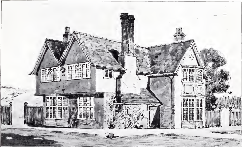
1614. House at Marine Parade, Gorleston-on-Sea, Norfolk, PAXTON WATSON, Architect.
